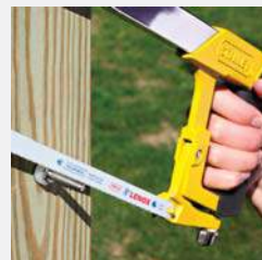
Step 2 Cut thread flush with nut.
