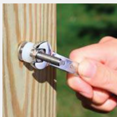
Step 1 Tighten nut to tension.
