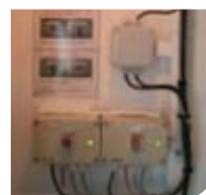
DEPLOYMENT PANEL FOR ACTIVATING MIS SYSTEM FROM EVACUATION STATION OR VESSEL BRIDGE
